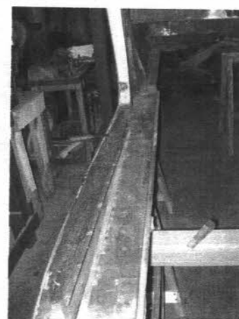
The original frame with badly damaged ends made a good pattern for the new frame
